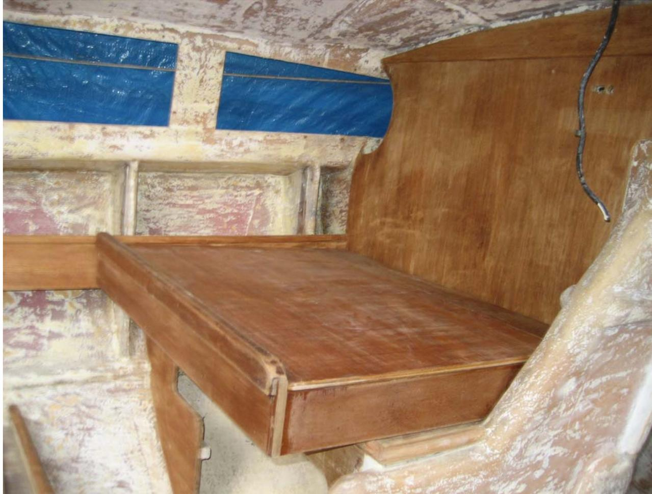
The original teak and mahogany internal bright-work is responding well to re-finishing and when varnished, together with white paint on cabin sides and keelbox will present an attractive traditional appearance.
